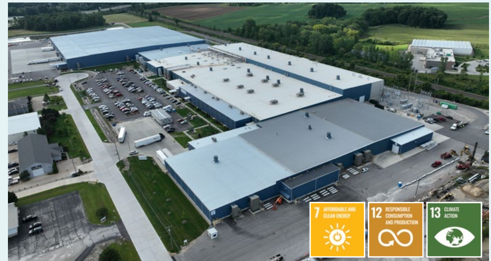
Ardagh Metal Packaging facility, Huron, Ohio
